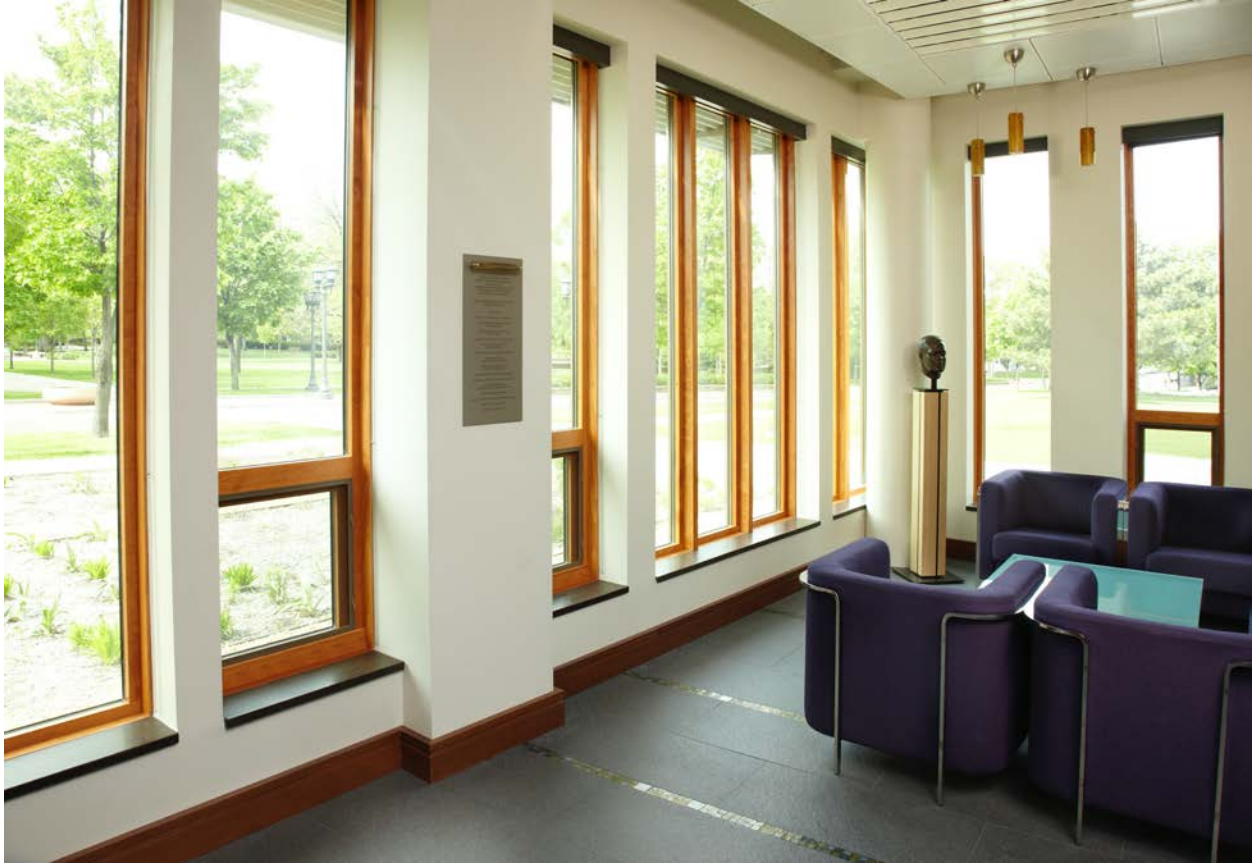
Stanley Shetka and Collateral Healing, Inc. designed, produced and installed all the Window Sills made in Markim Hall, made from 100% paper and plant byproducts
